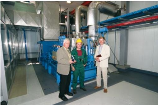
Turbogenerator 2,65 MW
